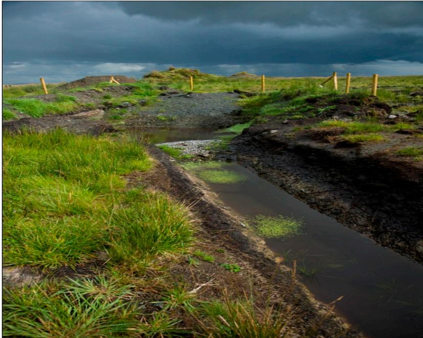
**Figure 4-2:** *Swale draining to Settlement pond*
