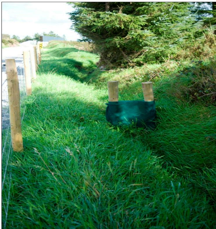
Figure 4-4: *Silt Trap across Grassed Swale*
