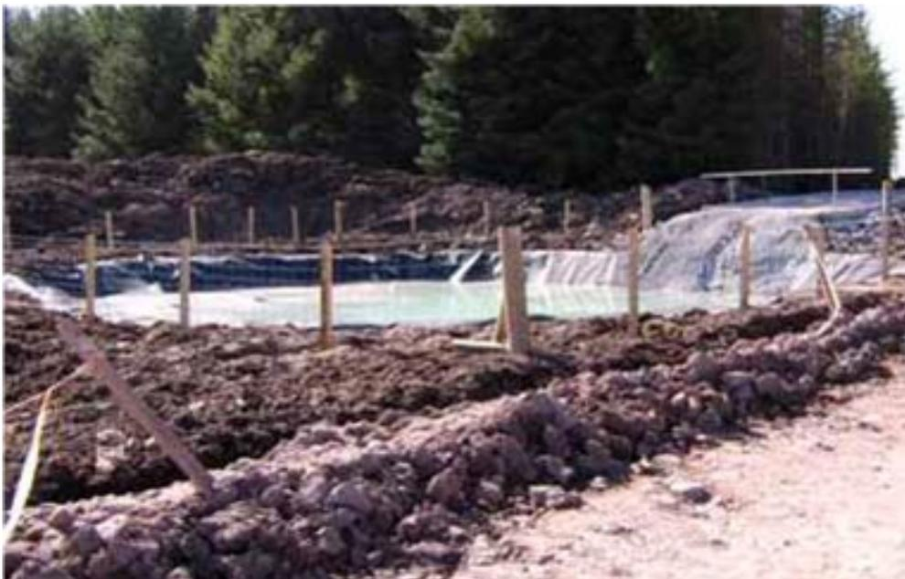
**Figure 4-8:** *Lined Settlement Lagoon for Concrete Washout Facility*
