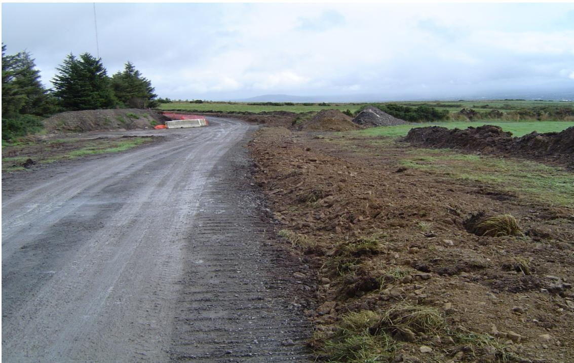
**Figure 4-7:** *Backfill over Cable Trench*
